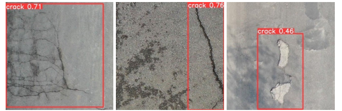
Fig. 19. Crack detection performance on asphalt pavement scene.
